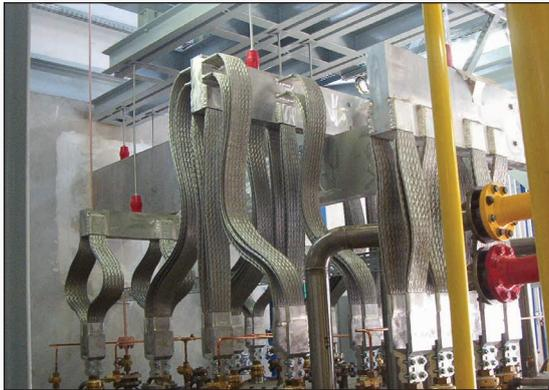
**Specific electrical connections** designed for specific needs of industrial process. The choice of technology and material is adapted to each project, respecting existing constraints in case of improvement of an existing equipment:
