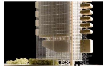
Figure 9 and 10 Lower screen and double facade of the San Paolo-Intesa Tower
